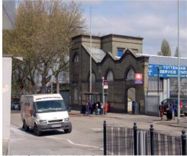
12. View along Tottenham Lane looking onto Hornsey Station
