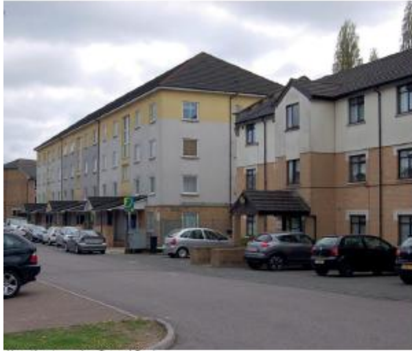
9. Varied housing stock on Denmark Road
