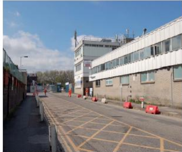
2. Looking towards the site along Hempsden Road with Willmott house on the right
